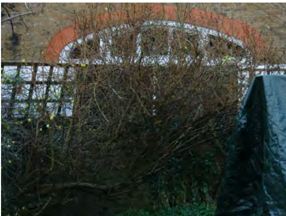
Picture 1.28 Central gauged red brick arch
