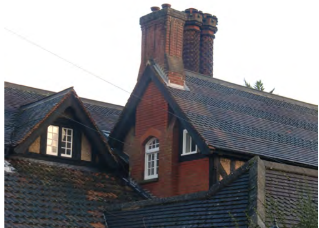
Picture 1.31 View towards attractive roofscape of locally listed 57 West Drive
