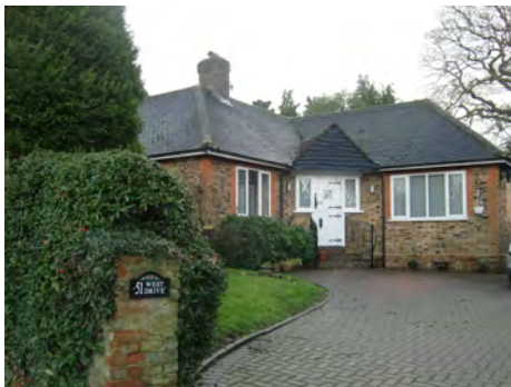
Picture 1.50 51 West Drive
