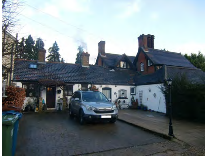
Picture 1.36 59 and 61 West Drive
