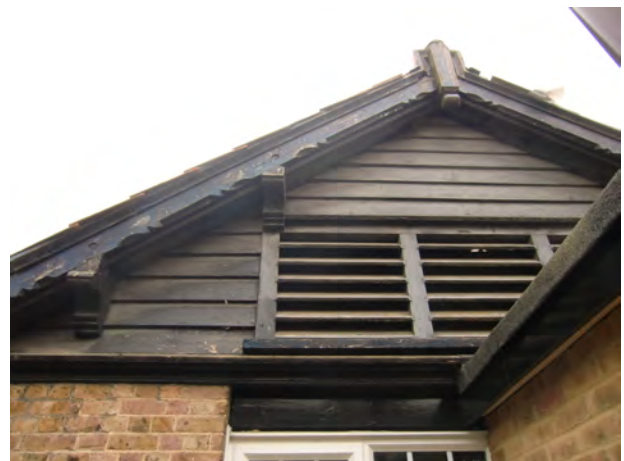
Picture 1.42 Original vents and bargeboarding to 40 West Drive
