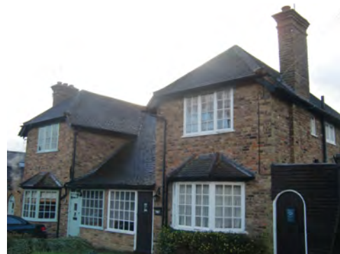
Picture 1.51 48 and 50 West Drive
