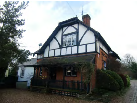
Picture 1.34 The former farmhouse - 47 West Drive
